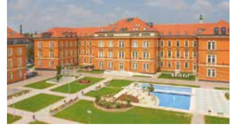
Project name: Leier City Center Location: Győr, Hungary
