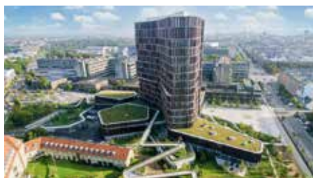
Project name: Panum Institute Location: Copenhagen
