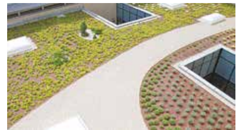
Project name: KÉSZ Office Building Location: Budapest, Hungary
